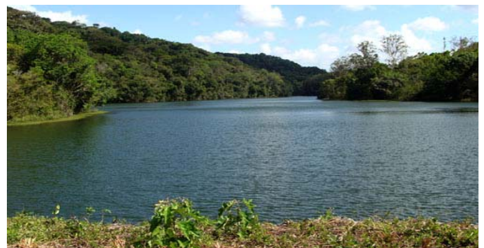
1d Weir located at USJ- Usina São José
